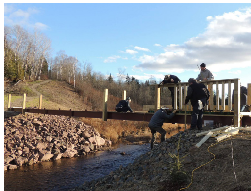
Volunteers working hard on the bridge. (Photo credit: Ray Riddell)
