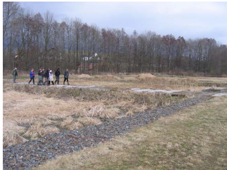
Participants inspecting a reed-bed sewage treatment area which treats the effluent from a town of 2,000, operated by the local land trust. (Stojan R.)
